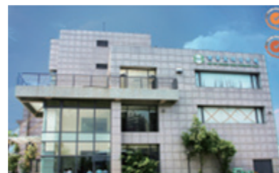
▼ Kaotan High-End-Water Purification Plant 拷潭淨水廠
